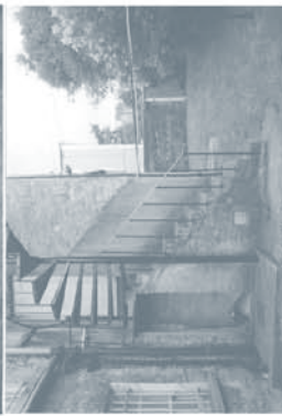
Side and rear external stone walls and cast iron fire stairs.
